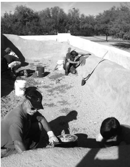
Pueblo Grande Mudslingers repair walls in lower rooms.
