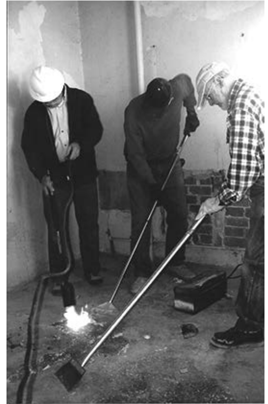
Ed Mack, Dick Myers and KJ Schroeder using a torch to remove linoleum at a January work day.
