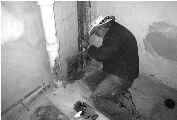
Wilson Allen patches a wall at Toltec School
