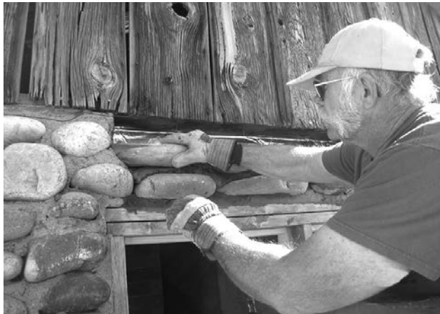
KJ Schroder reconstructing cobble wall above window.
