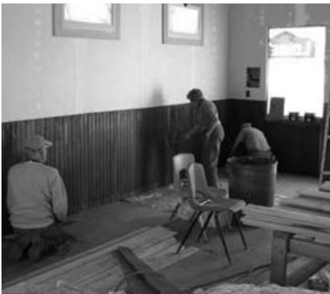
SWAT members staining beadboard siding.
